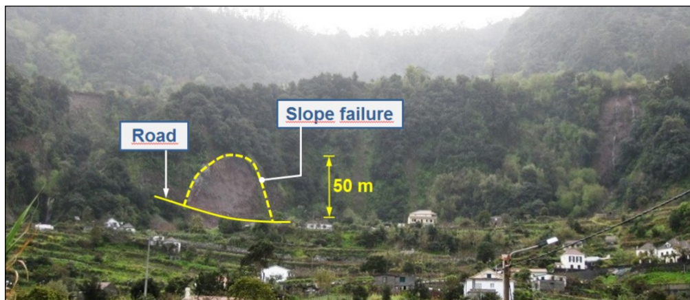
Figure 17. Slope failure close to the village of Arco de São Jorge.
