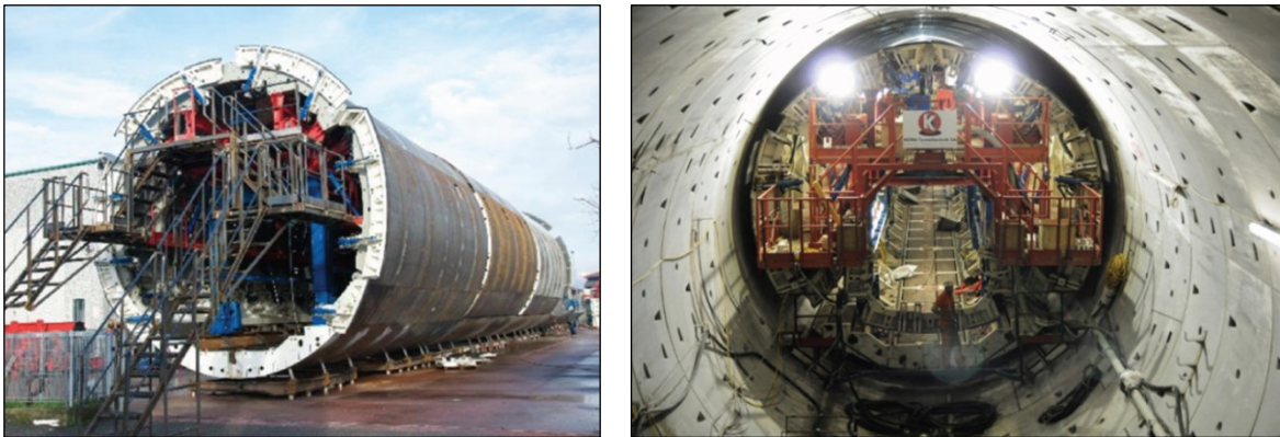
Figure 16. Secondary tunnel lining.
