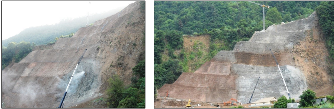
Figure 18. Slope stabilisation works.
