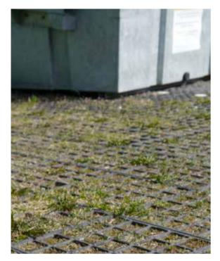
Since more than 20 years PURUS PLASTICS manufactures the ECORASTER® permeable ground reinforcement system, made of recycled materials (LDPE). For about the same amount of time the very first ECORASTER® E50 "classic" is installed at a highly used waste collection point. Although there are lots of heavy switching moves and loads caused by the lifting and setting of the containers the area is free from settlements, edges and ditches. In the meantime the area got greened spontaneously.
